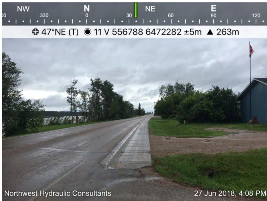
View looking downstream along River Road at the Water Survey of Canada gauging station (the Legion building is on the far right)
